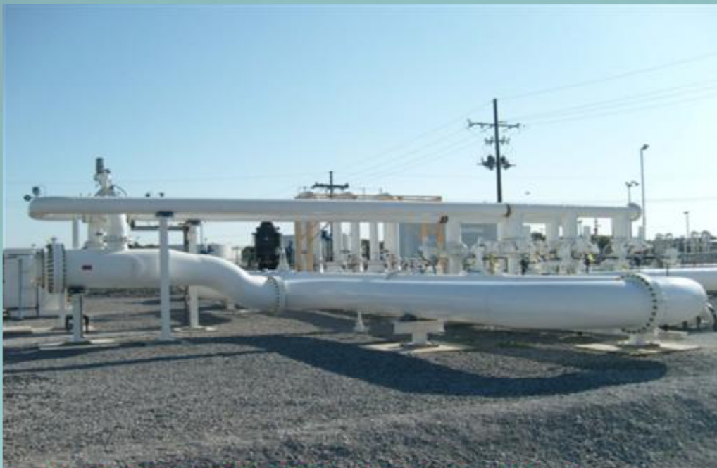
Pipeline & Meter Station Project (Gibson, Louisiana)
